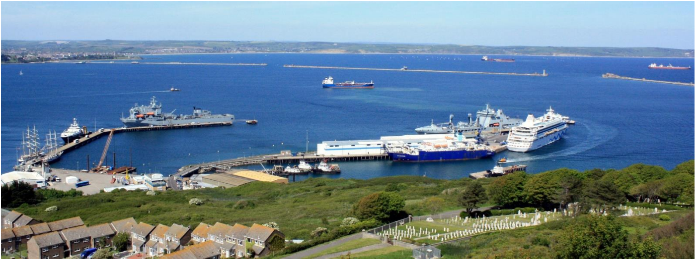
P1 Portland Port May 2019
